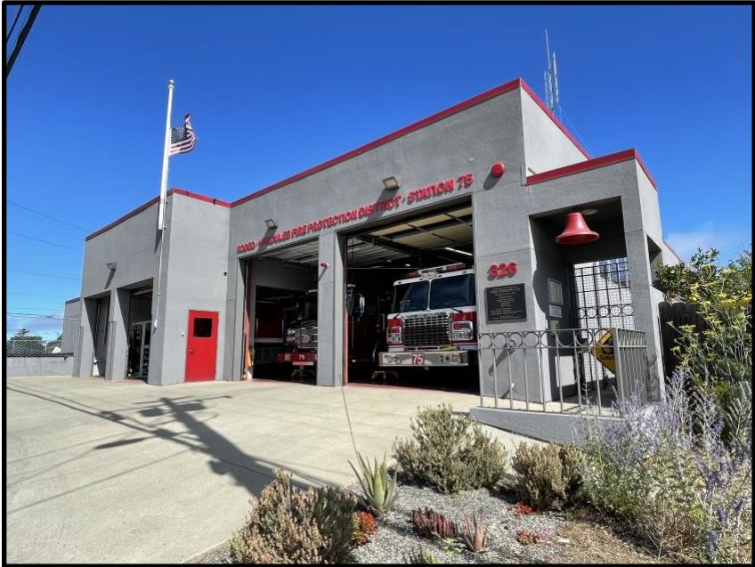
Station 75 - 326 Third Street. Rodeo, CA 94572
